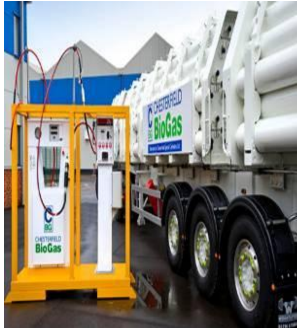
(b) Biogas dispensing station with bulk cascade of cylinders in UK (Source: http://www.chesterfieldbiogas.co.uk/news/Chesterfield-BioGas-trailer-fuels-Coca-Cola-Enterprises-supply-vehicles/6 )
