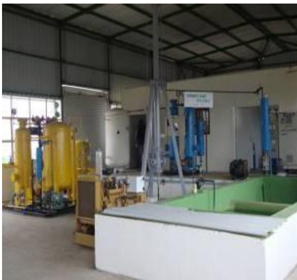
(a) Water scrubbing and PSA system
