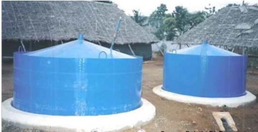
Figure A4. Community biogas plant (Source: http://balajibiopower.com/ )
