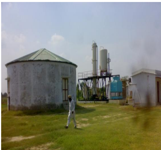
(a) Biogas Plant
