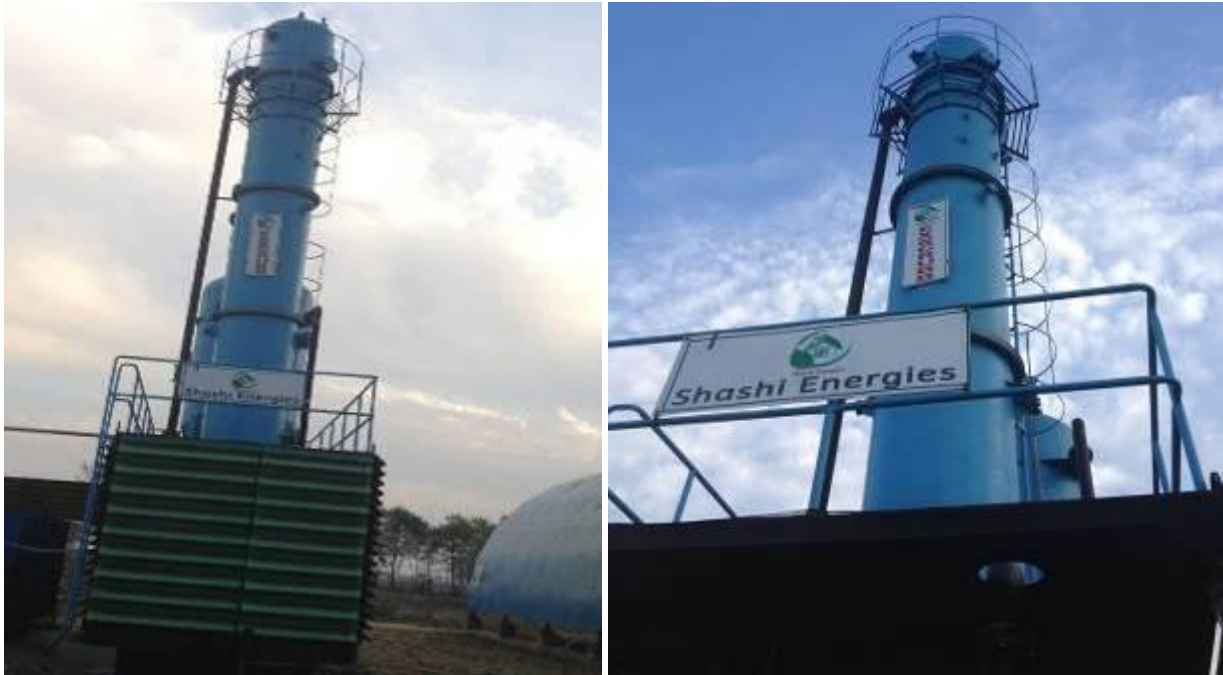
(a) and (b) 50 \text{ m}^3 \text{ hour}^{-1} Low Pressure Water Scrubbing Tower
