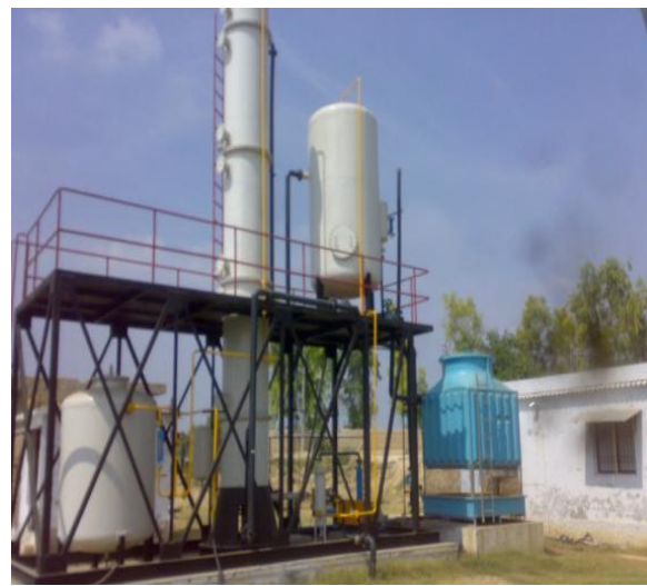
(b) Upgrading Plant
